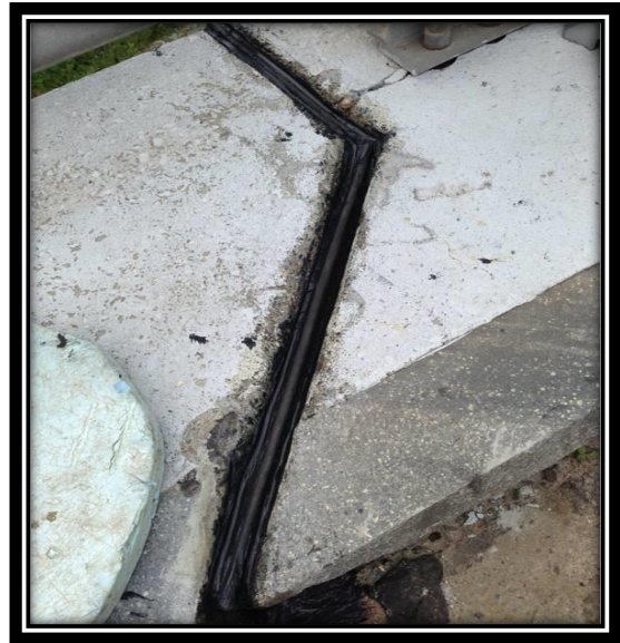
SF225 Gland Spliced to Accommodate a Skew
