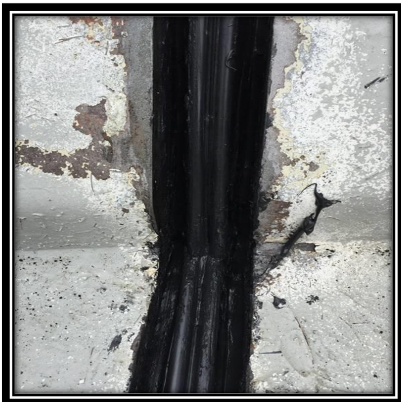
SF400 Gland Spliced to Turn Up a Barrier Wall
