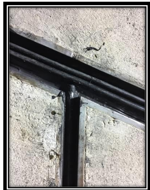
SF225 Gland "Tee-Spliced" into SF400 Gland
